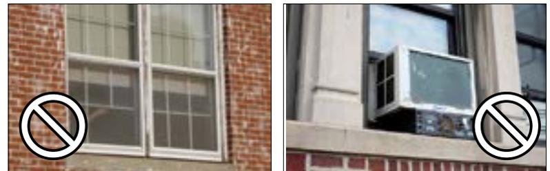
(right) Window AC units cause a visual impact, put weight on window units and often drip condensation on sills. (Left) Modern vinyl replacement windows (when installed rated higher than the existing 50-year wood windows they replaced). Only 15 years later the "grid-between-glass" mullions are dropping, parts have shrunk and visual character does not match.
