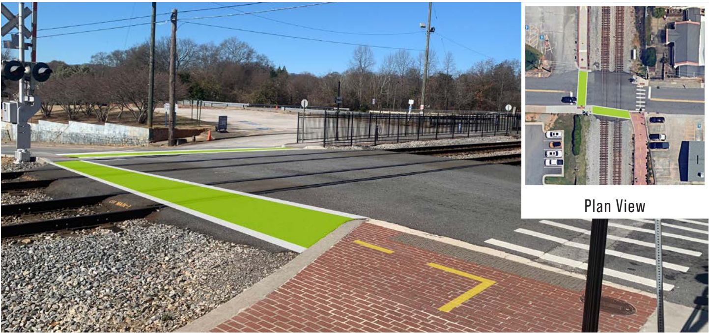
Solid color painted crosswalk with dashed median lines.
