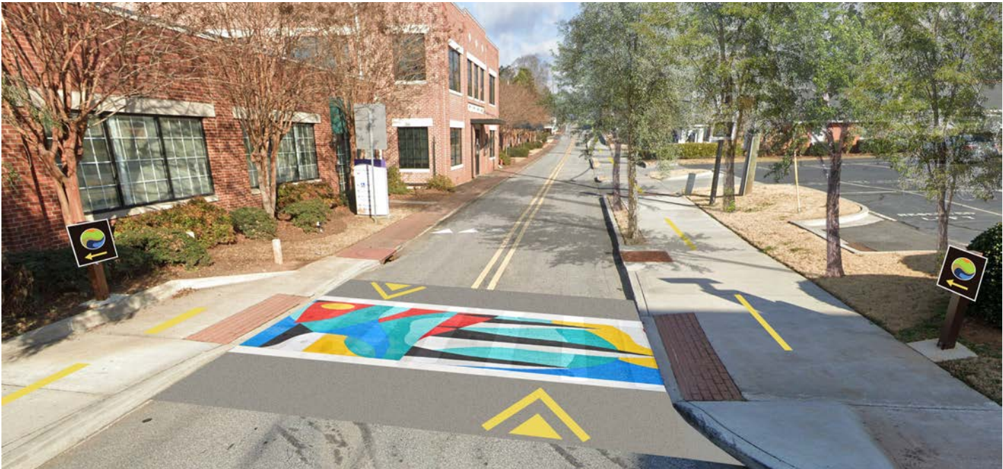
Artistic crosswalk design, raised crosswalk, dashed median markings on the trail path, more obvious trail signs at both sides of the street, and street trees in the planting strips along the eastern side of Roselane St.
