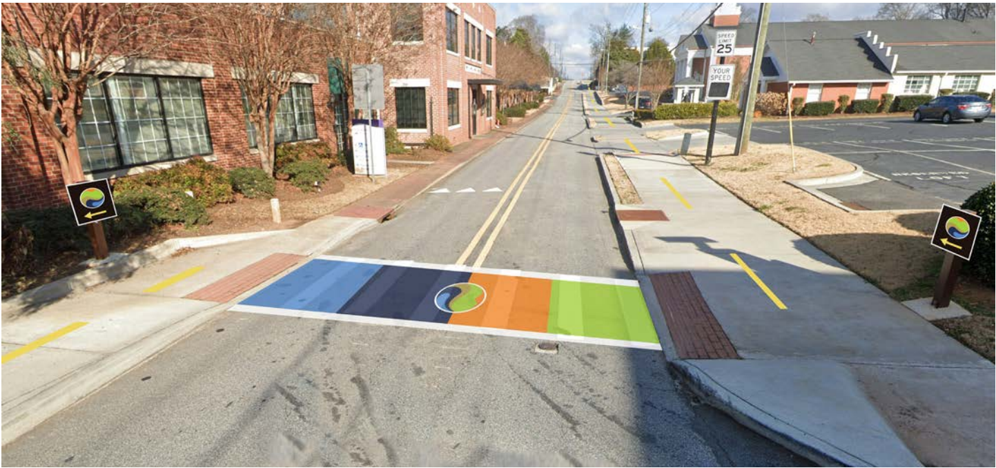
Painted crosswalk and dashed median markings, with more obvious trail signs at both sides of the street.
