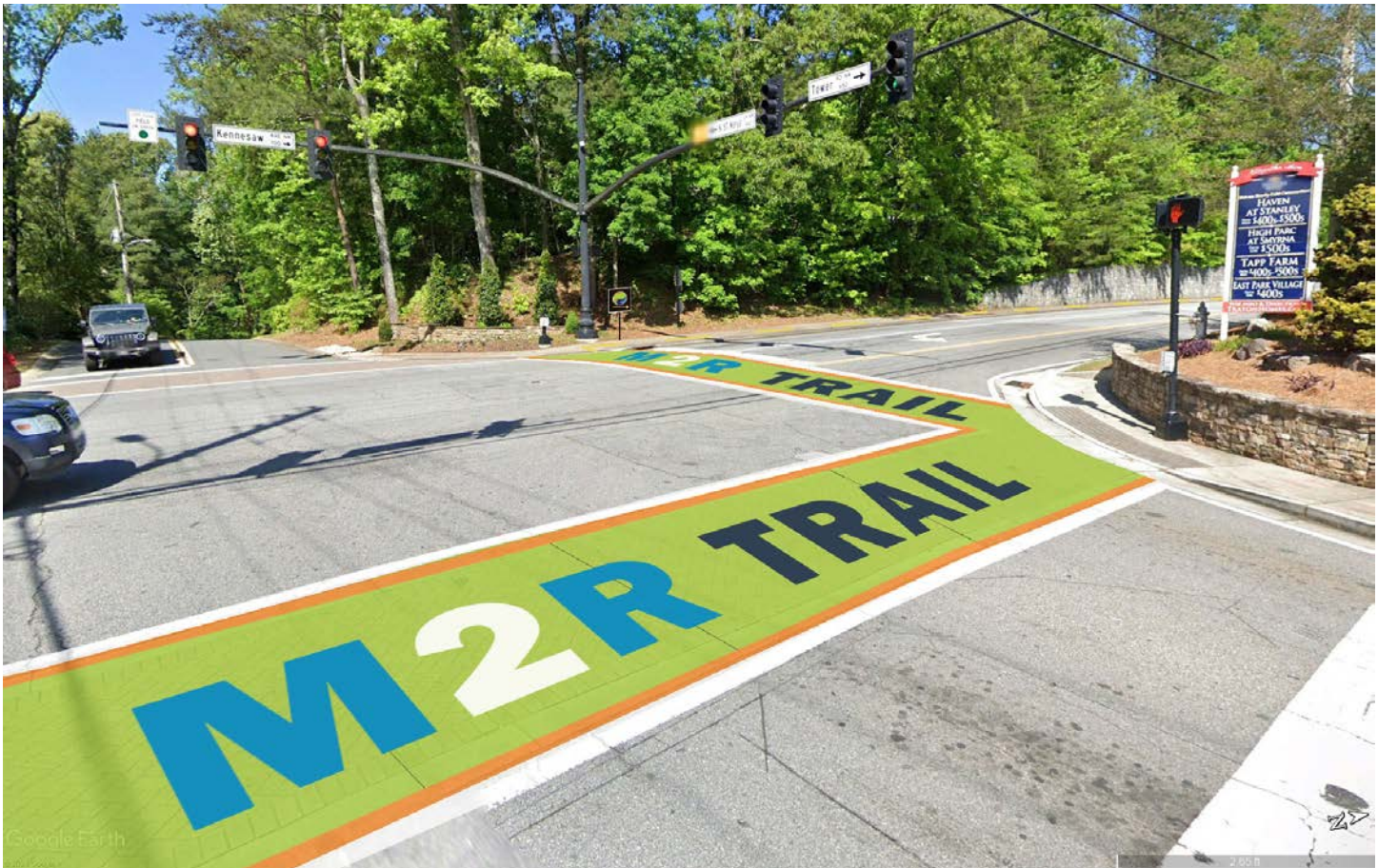
Painted crosswalks with the name of the trail integrated into the crosswalk design, a sign at the far corner visible to northbound users (across the street), and dashed median trail markings (across the street) continuing up Kennesaw Ave.
