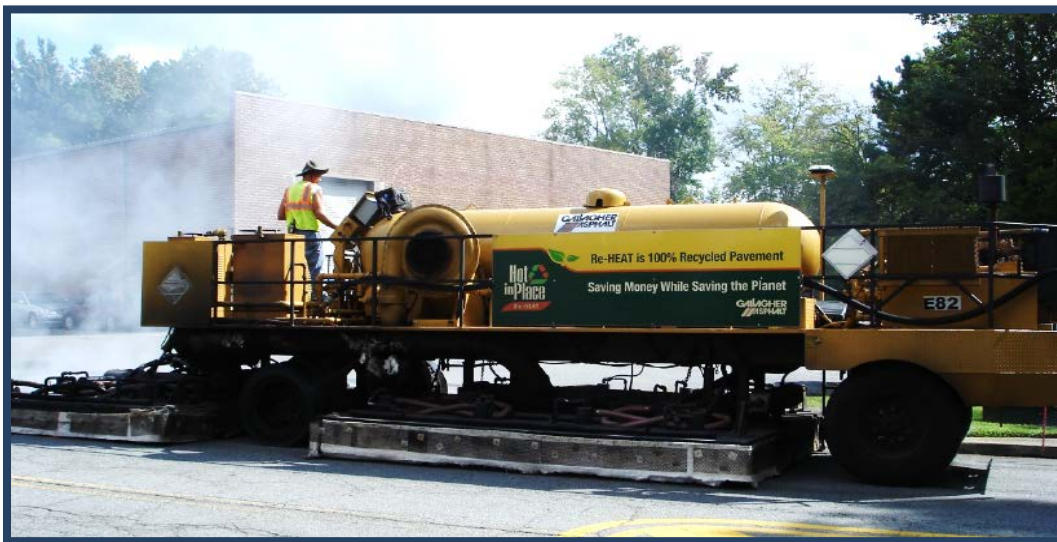
Annual Street Resurfacing - Streets resurfaced by Re-HEAT 100% Recycled Paving
